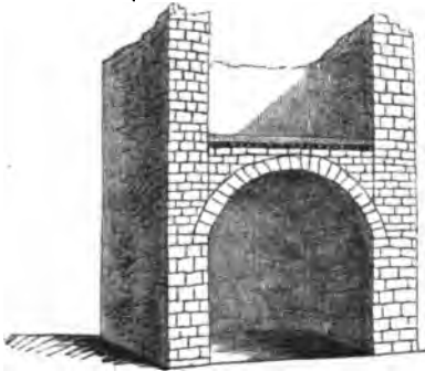
No. 129. Flooring over an arched room. Thebes.
